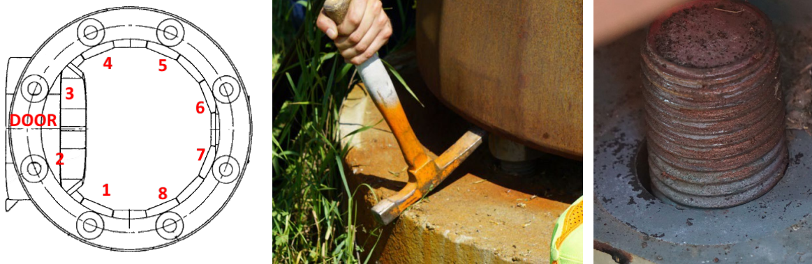
Figure 3.3.16. Rod numbering (left), checking washers for looseness (center), and prior copper anti seize lubrication on rod (right)
