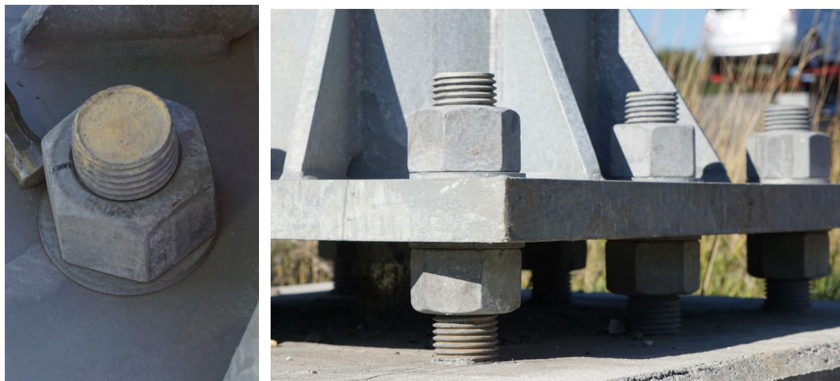
Figure 3.2.8. Turn-of-nut marks on nut (left) and baseplate of OH I-94-688 (right)
