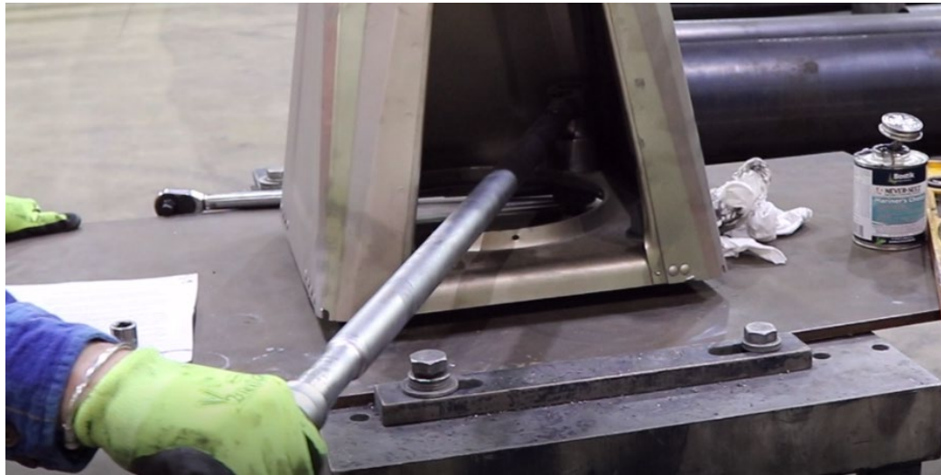
Figure 3.3.8. Final verification torque on the structure installation
