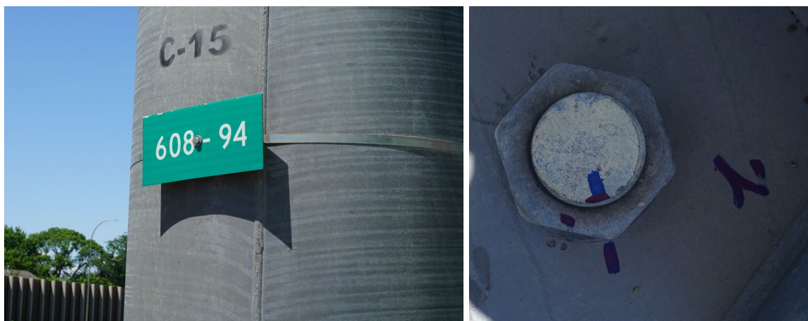
Figure 3.2.14. I-94-608 Post (left) and 1/12 turn on nut #8 (#2 in star pattern) (right)
