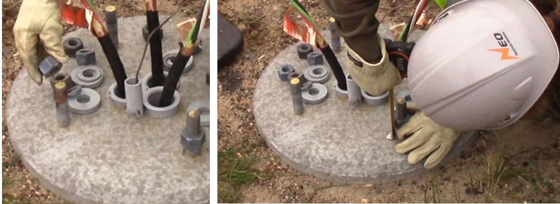
Figure 3.3.1. Placing leveling nuts (left) and verifying standoff distance (right)
