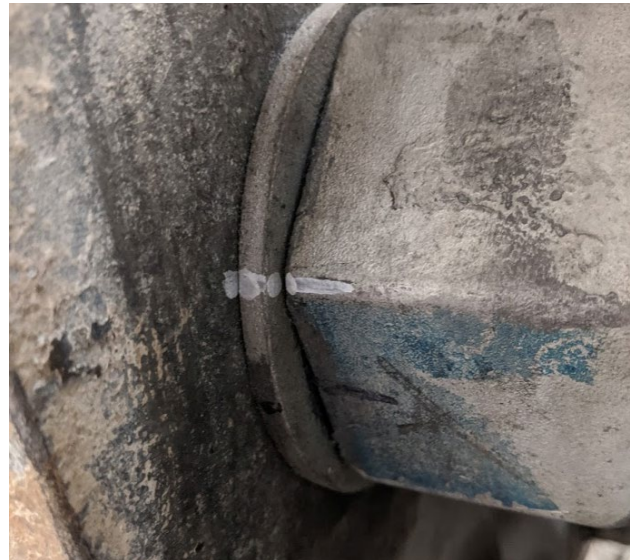
Figure 5.1.4 (Left): Example Turn Marks after Tightening on Top and (Right) Leveling Nuts
