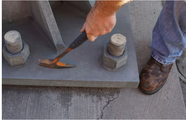
Figure 3.1.1. Checking for clamping force in connection
