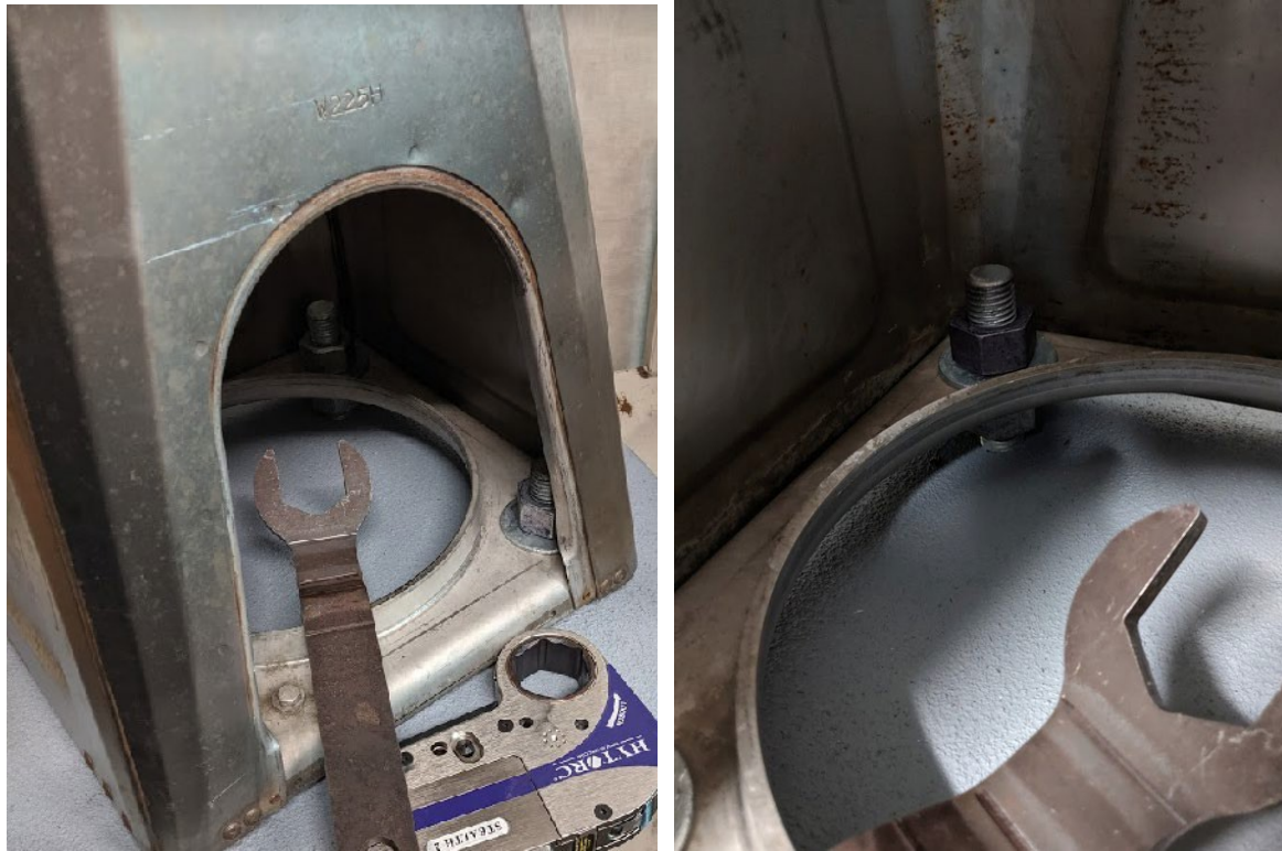
Figure 3.3.27: Exterior of Light Pole Base (Left) and Interior of base (Right)
