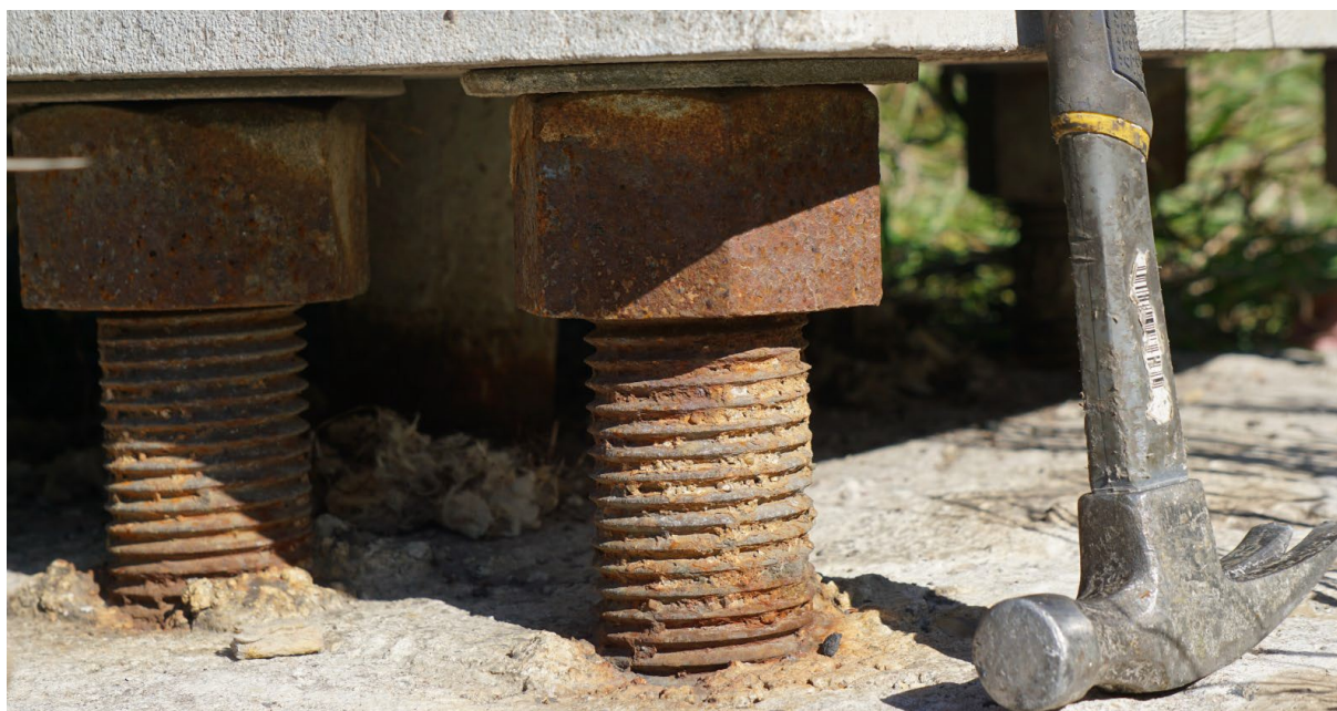
Figure 3.2.9. Large standoff distance on I-494-153 structure
