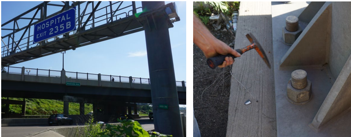
Figure 3.2.11. Full truss OH sign I-94-602 (left) and inspecting rod pre-tension force (right)
