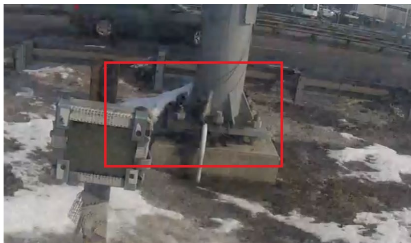
Figure 4.2.5. Snow and ice piled on anchor rod gauges
