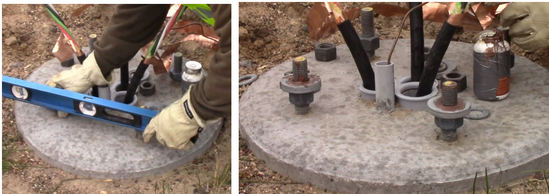
Figure 3.3.2. Leveling process (left) and improper lubrication of leveling nuts (right)
