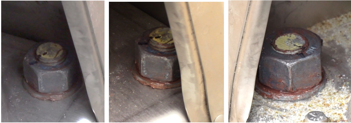
Figure 3.3.4. Nut turns at initial, second step, and final values (left to right)
