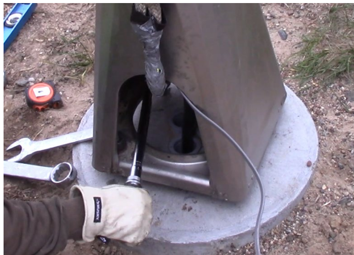
Figure 3.3.5. Applying verification torque
